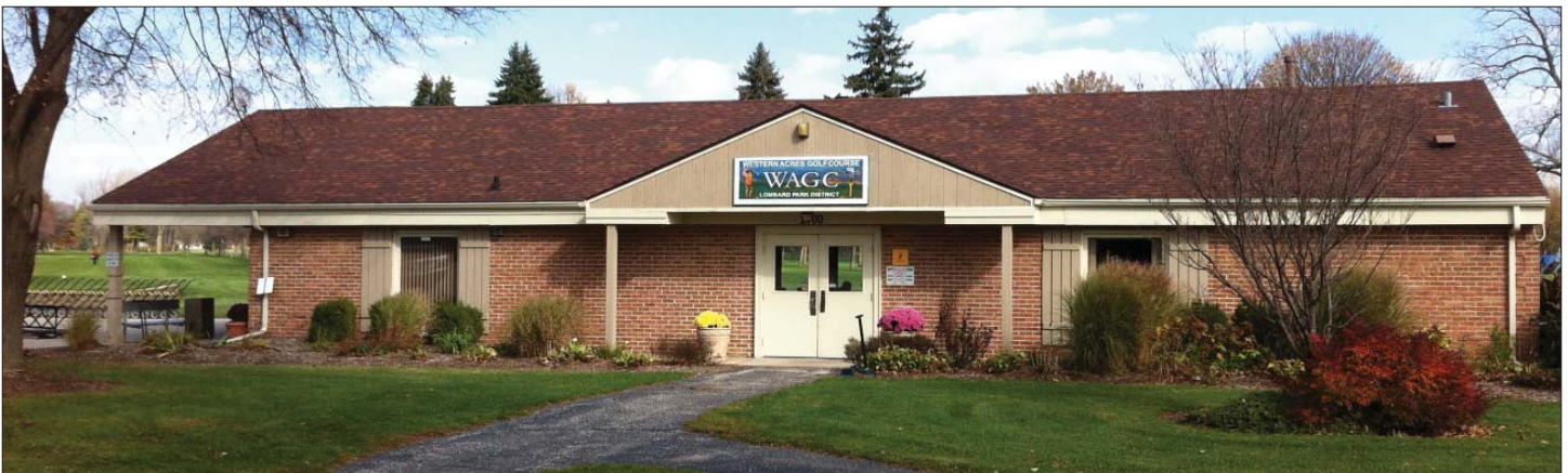
Front View of Building
