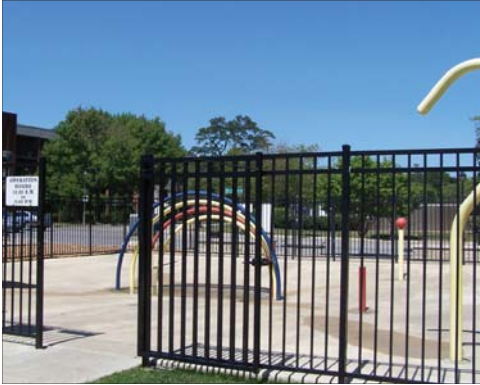
Entry Gate for Spray Park
