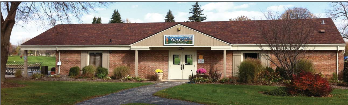
Front View of Building
