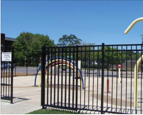
Entry Gate for Spray Park
