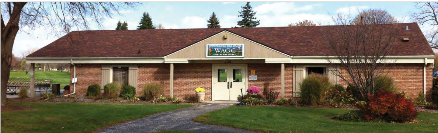
Front View of Building
