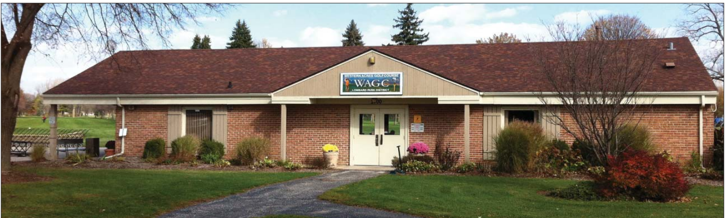
Front View of Building
