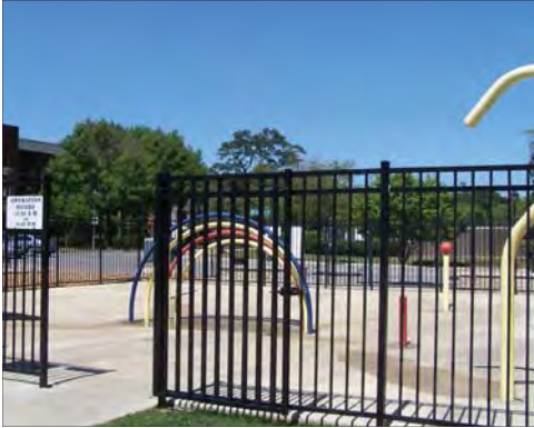
Entry Gate for Spray Park
