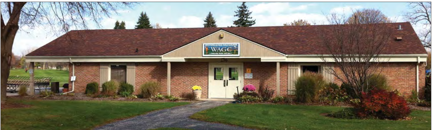
Front View of Building
