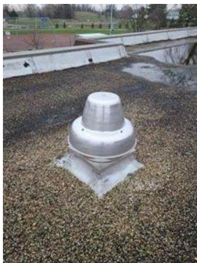
51. Roof Exhaust Fan (typical)
