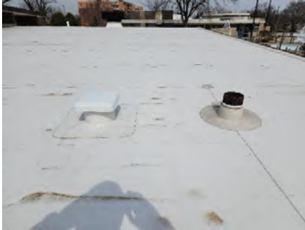
16. Low exhaust fan and pipe penetrations
