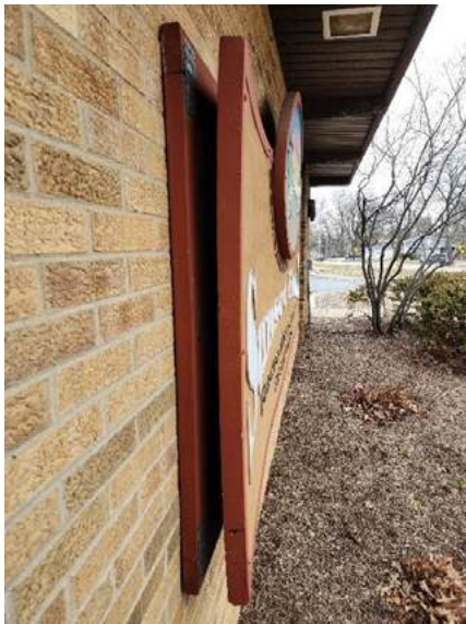
17. Building sign warped away from building
