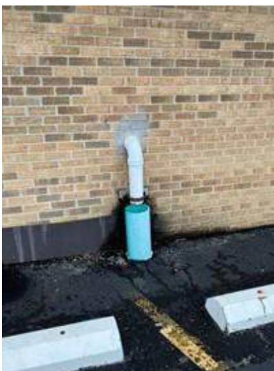
54. PVC Storm Piping to Sewer
