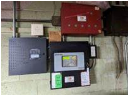
105. Existing Fire Alarm Panel
