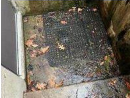
35. Drain at Basement Landing
