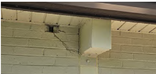
9. Stepped cracking at brick masonry veneer wall
