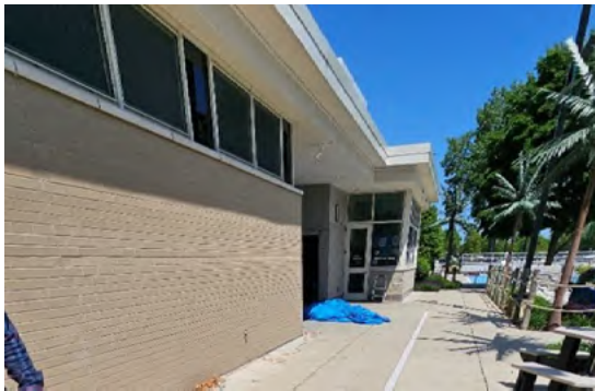
11. Brick veneer façade with storefront glazing system
