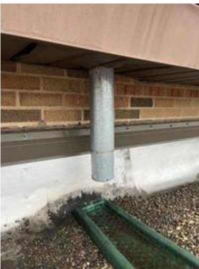
66. Multi-purpose Roof Drain to the Main Roof
