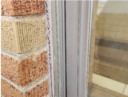
10. Sealant at window jamb
