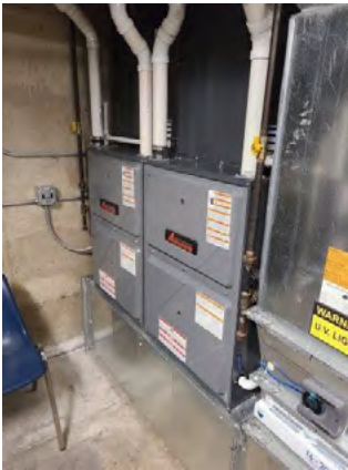
28. Gas-fired Furnaces (typical)
