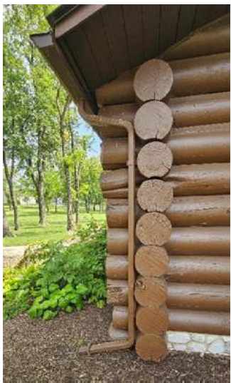
12. Roof gutter and downspout
