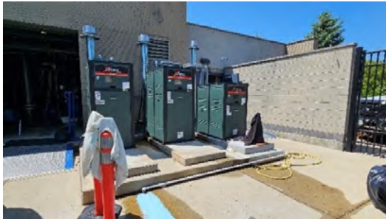
31. Exterior storage area, condensing pool heaters
