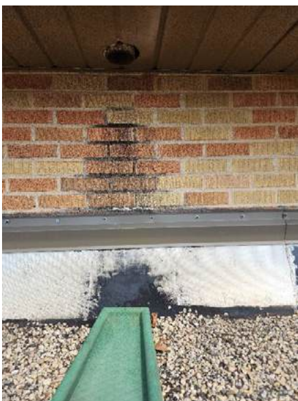
24. Upper roof downspout thru soffit
