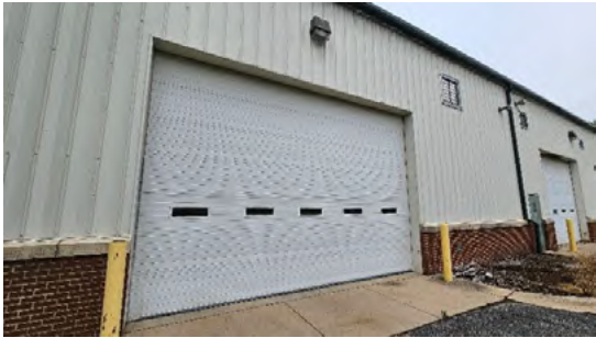
8. Operable mechanical coiling doors access
