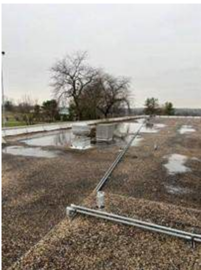
57. Ponding on Roof
