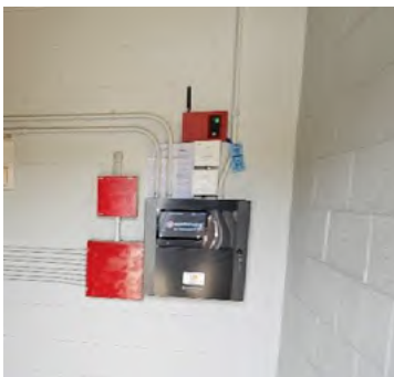
33. Fire alarm system at sprinkler room
