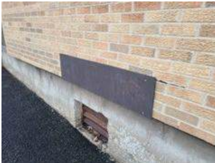
46. Covered Unit Ventilator Air Louver
