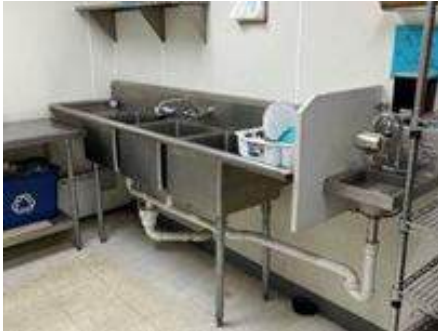
76. Three-compartment Sink
