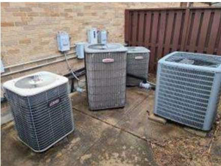
29. Air-cooled Condensers (typical)
