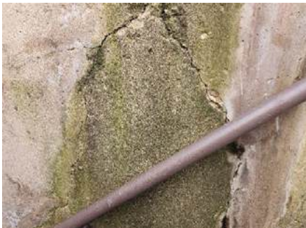
15. Cracks in stair wall
