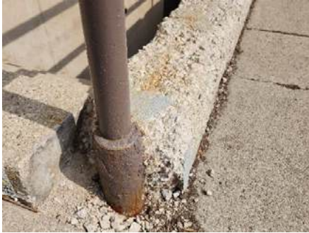
13. Crumbling concrete at top of stairs
