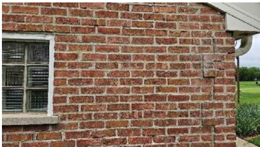
8. stepped cracking along brick facade
