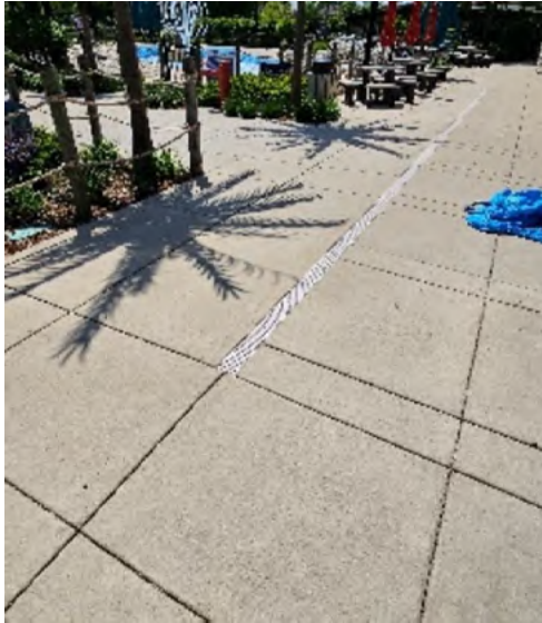
4. Site hardscape at linear area drain
