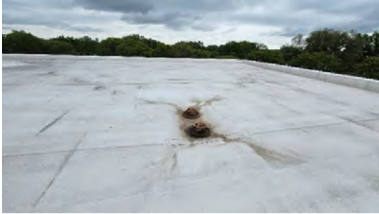
10. Roof slope to area roof drains
