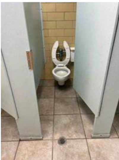
69. Water Closet and Floor Drain
