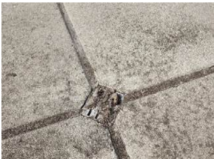
9. Blocked sidewalk drain
