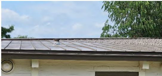
10. Existing standing seam metal roofing system
