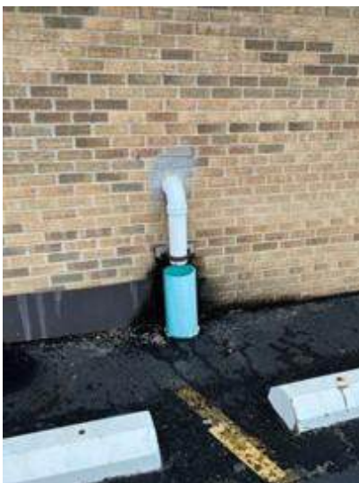
63. PVC Storm Piping to Sewer
