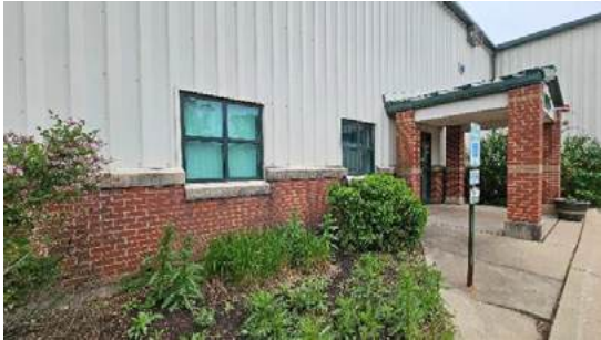
7. Prefabricated metal façade with brick veneer
