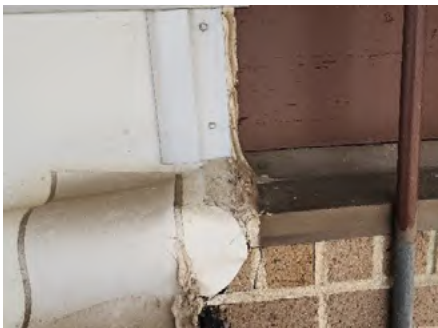
17. Lower roof edge to wall condition
