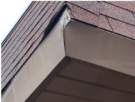
19. Asphalt shingle outside corner
