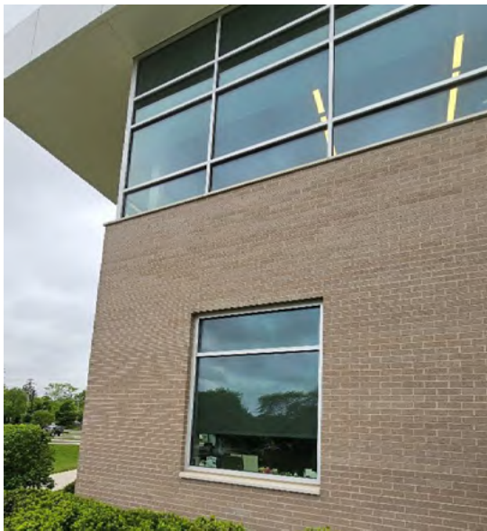
8. Punched window opening and storefront glazing
