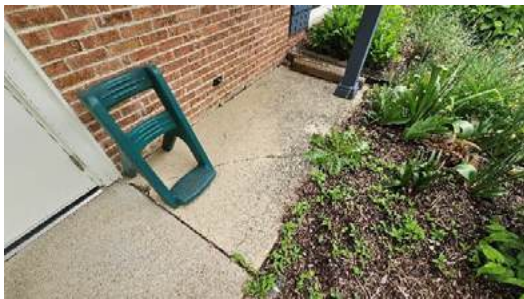
6. Visible cracks at concrete entry sidewalk
