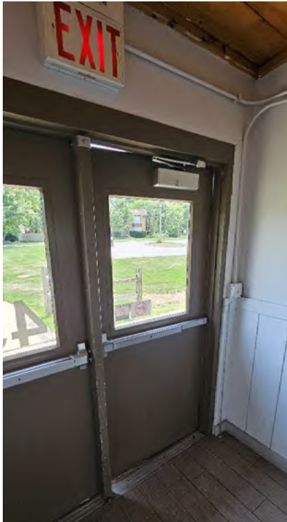
13. Main entry double door with panic hardware
