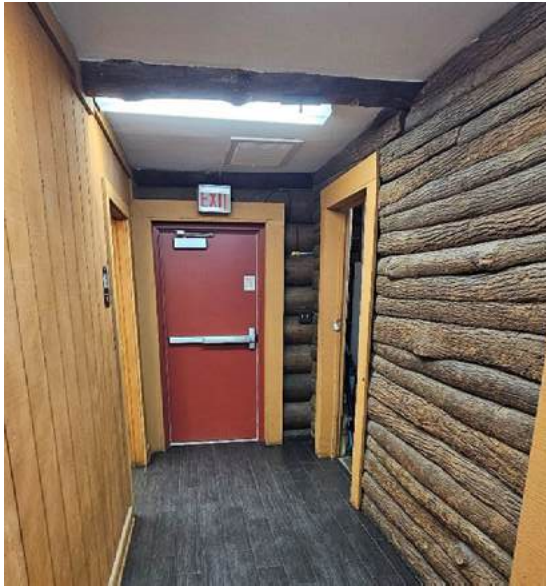
13. Main entry door access with panic hardware
