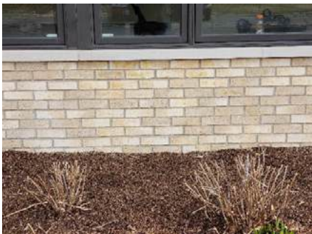
12. Efflorescence on brick
