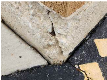
18. Cracked foundation at outside corner
