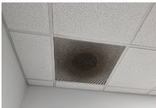
30. Return air grilles, dirt and debris within grille, typical
