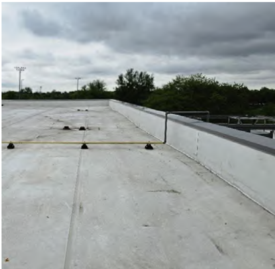
12. TPO membrane at roof and parapet wall.
