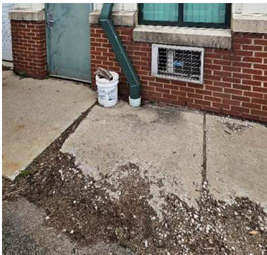
6. Degraded concrete pads and walkways
