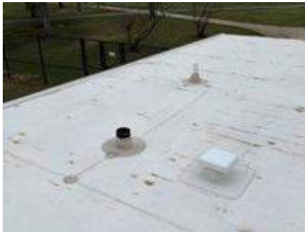
30. Cast Iron and PVC vent thru roof
