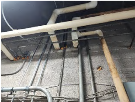
40. Boiler room penetrations
