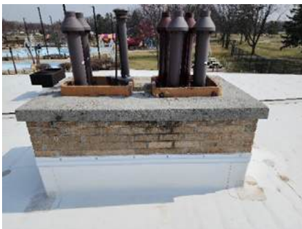
18. Old chimney with new pipes thru
