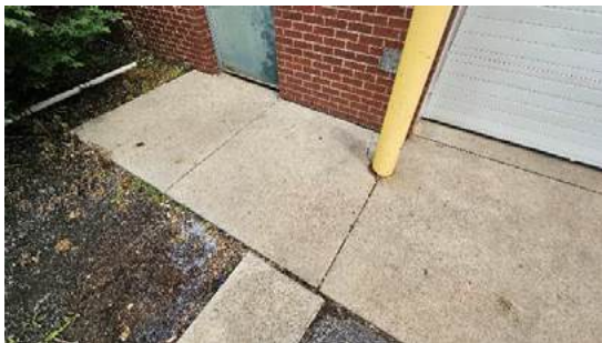
5. Cracking present at concrete entry pads and walkways
