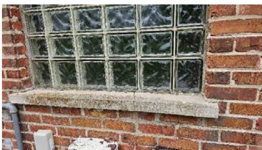
9. Stone windowsill cracking present
