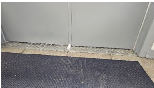
14. Exterior entry doors, visible light gap between doors
