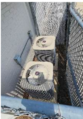
22. Air conditioner condenser units
