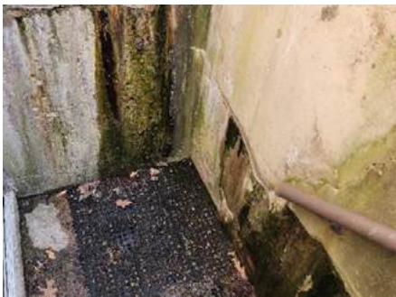
14. Water and algae growth. Blocked drain
