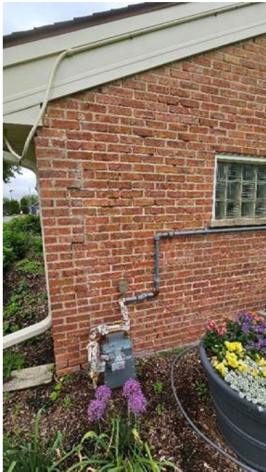
7. Inconsistent and visibly deficient mortar joints
