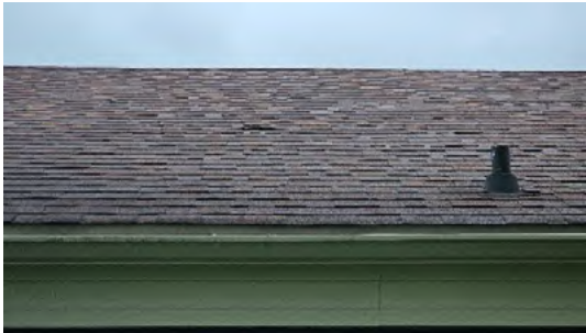
10. Asphalt shingle roof, shingle uplifted
