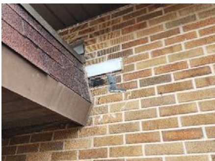
12. Tar and staining on brick veneer
