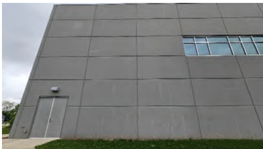
9. Exterior architectural precast concrete system
