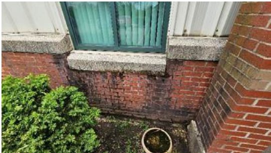
9. Damage at brick veneer facades
